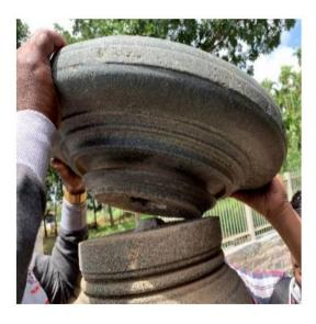
Figure 12: Tabled joint in the columns
