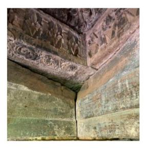
Figure 17: Missing clamps at beam connections
