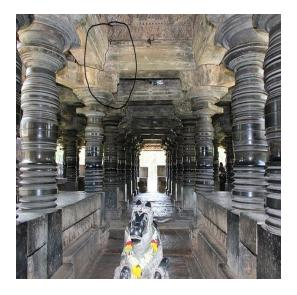
Figure 5: Cracks and chipping of stone at the beam-column joints
