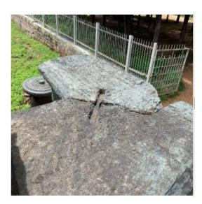
Figure 13: Cramped joint used in the beam connections
